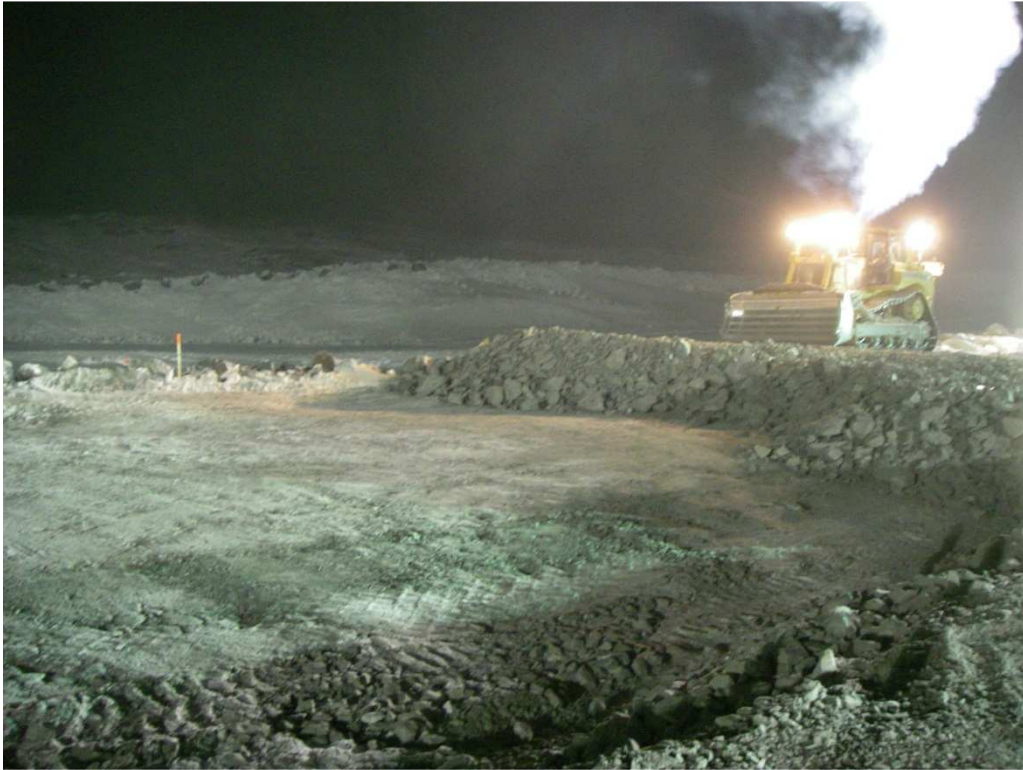
Photo 8: CAT D8 dozer placing ROQ on the downstream of the dam.
