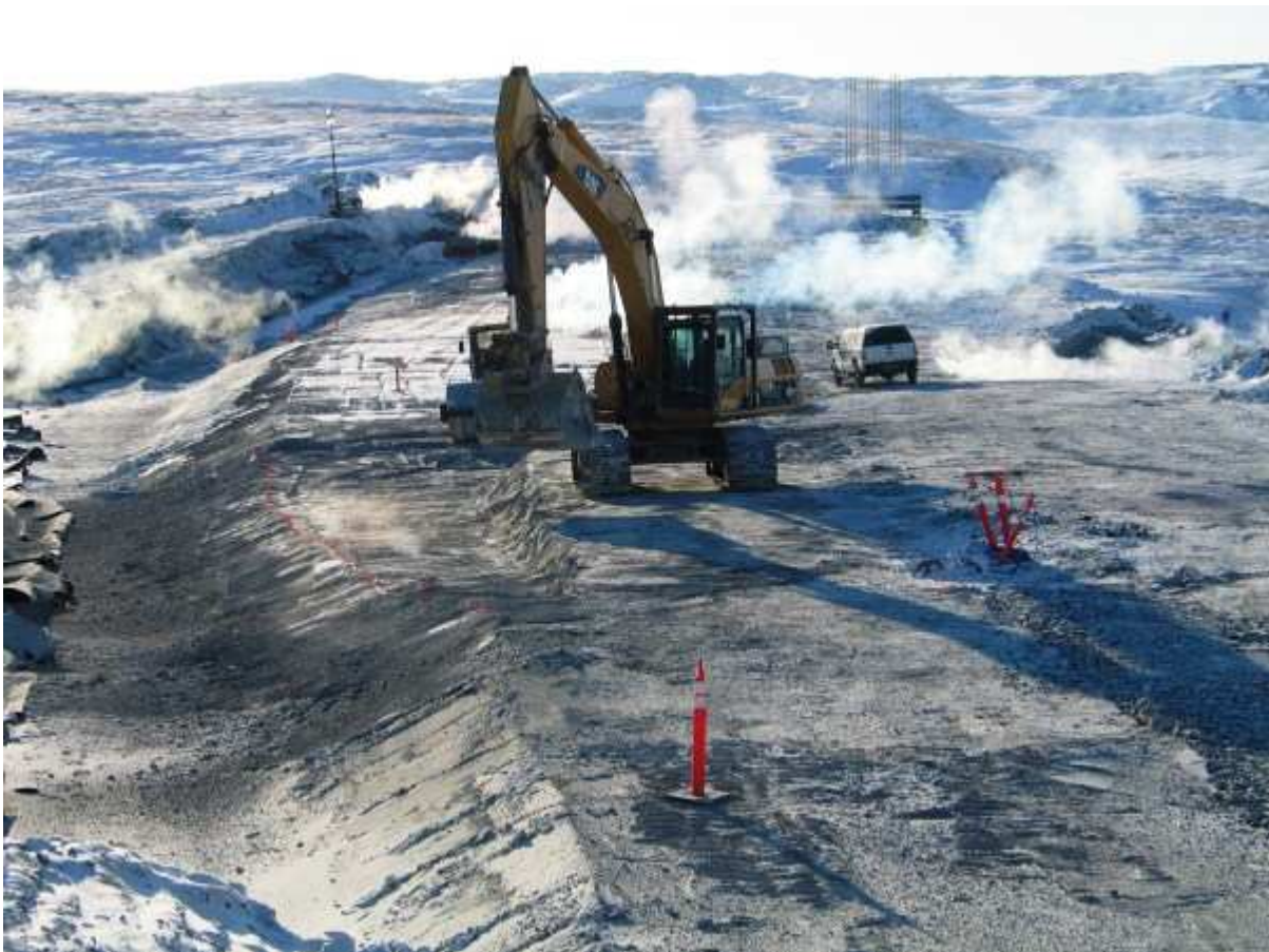
Photo 7: Work area cleaned prior to placing FCM.
